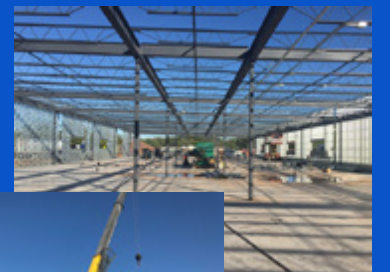
Bonham Elementary Construction
